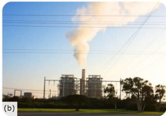
(b) A small coal-fired power plant.
